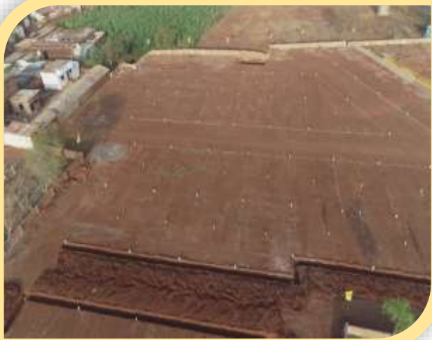
Nisarga Gurudwara Phase2 Plotting Project. Land Area 18.52 Acres. NA&Buda Approved Project
