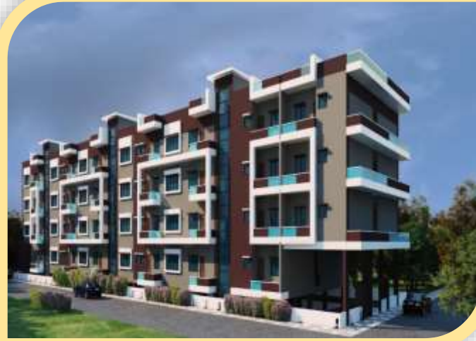
Nisarga Gurudwara Apartment Project. NA&Buda Approved Project
